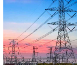
POWER GENERATION & TRANSMISSION
